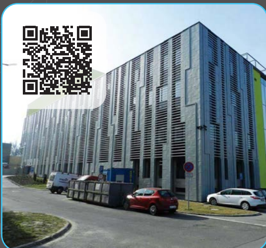
National Supercomputing Centre Ostrava
