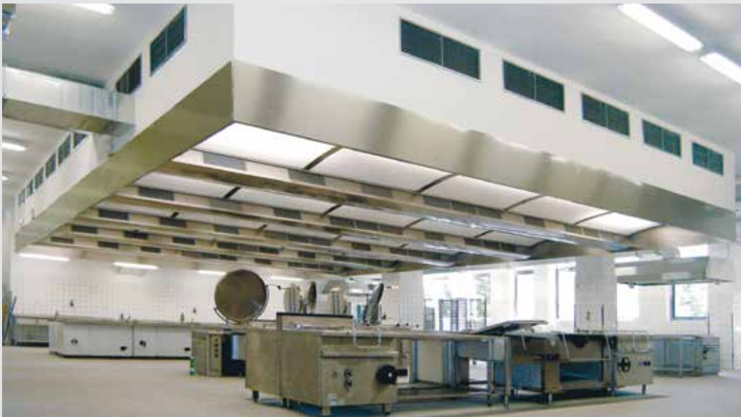
Army catering facility Vyškov
