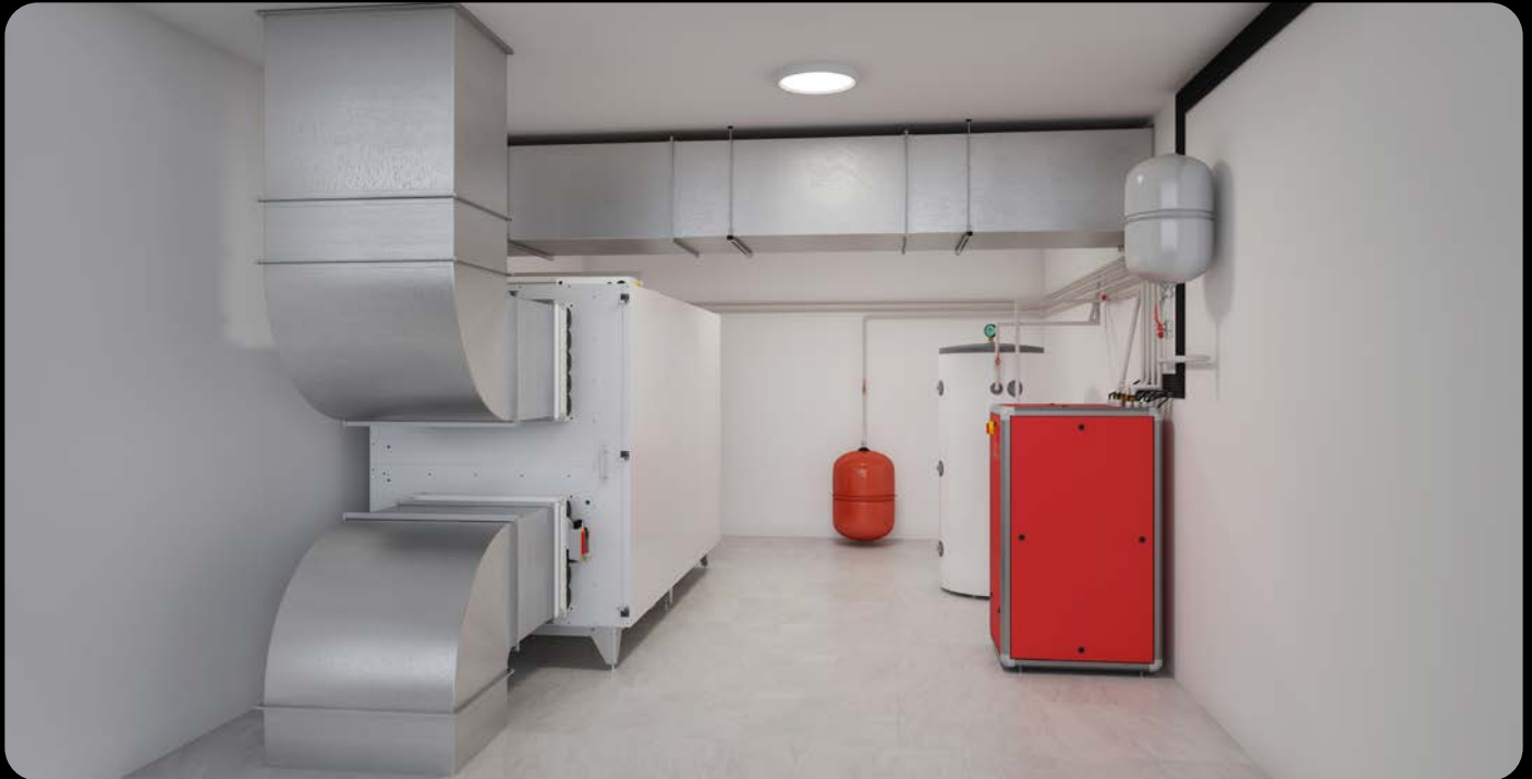
Sample utility room with a DUPLEX Basic 15100 ventilation unit with heat recovery, a MasterTherm AQ90I heat pump and a heat storage tank.
